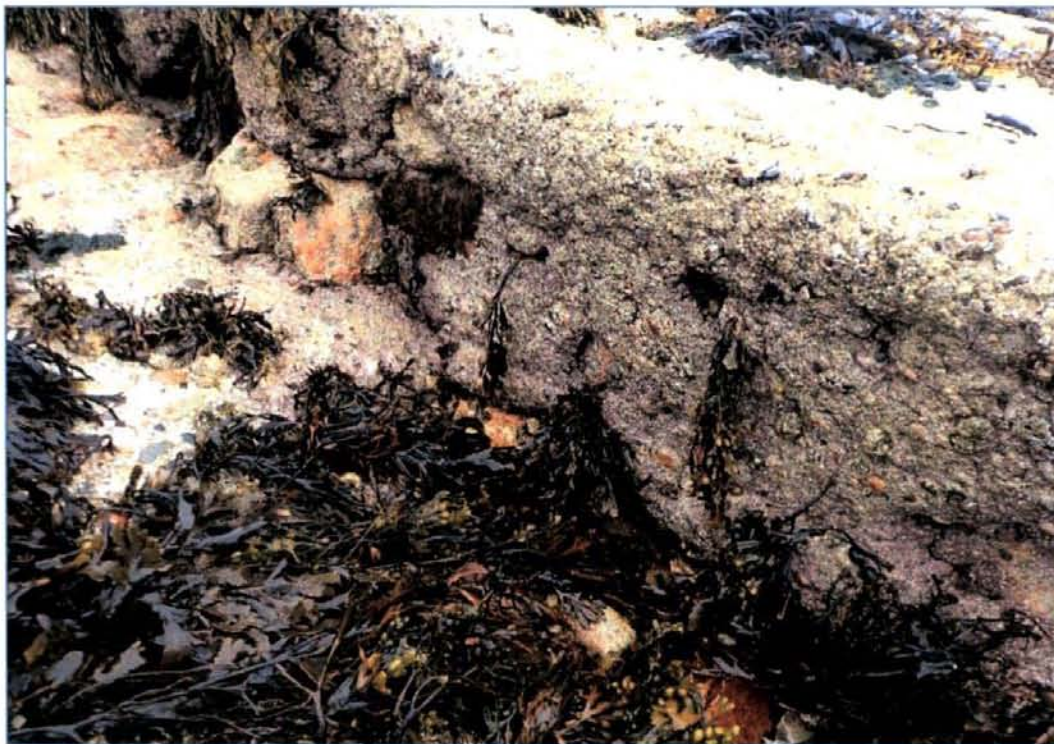
Plate 40: View of side of slipway, showing its construction using unshaped stone bedded in mortar.
