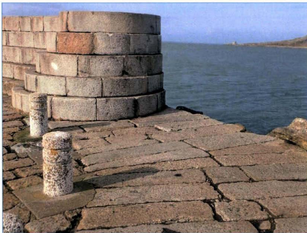
Plate 19: The stepped granite ashlar wave barrier at the West Pier roundel.
