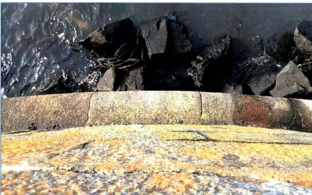
Plate 22: View from above looking down on rolled moulding on exterior of West Pier roundel.
