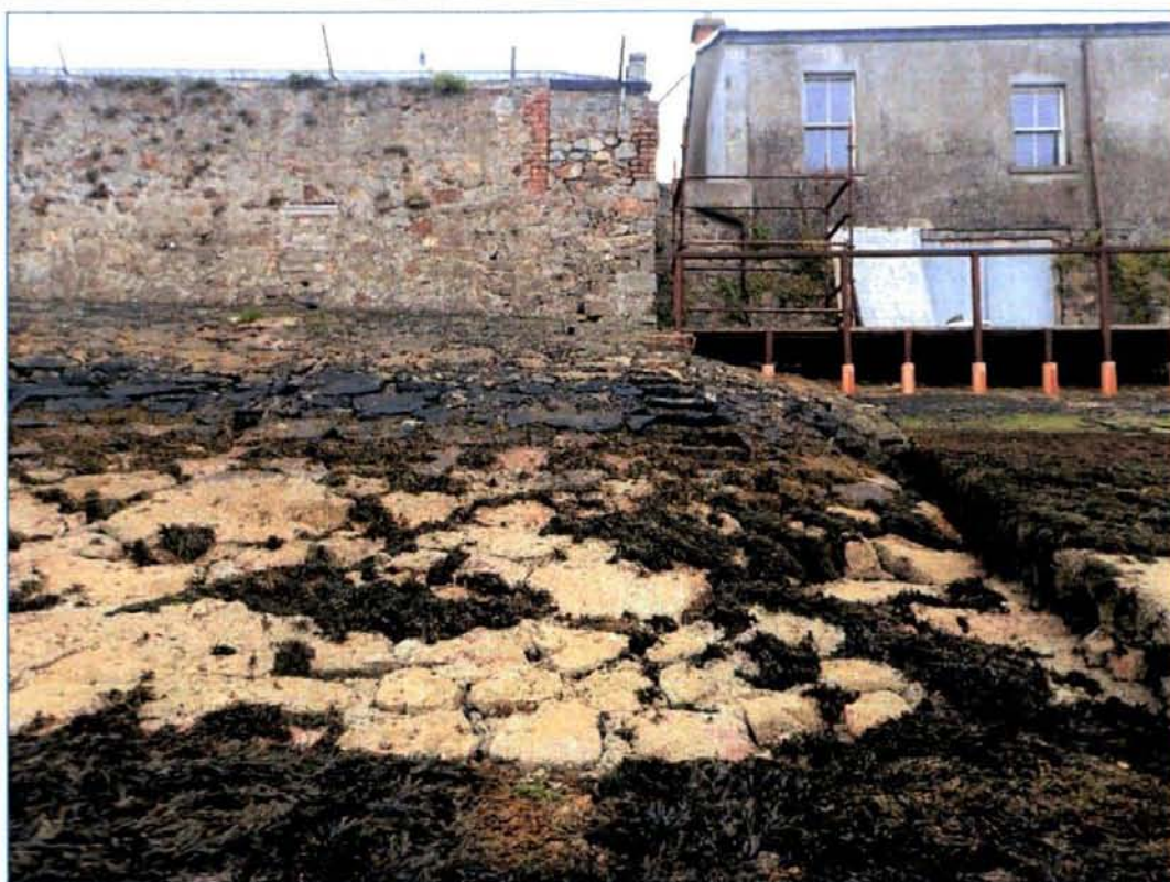
Plate 38: Close-up view of rear of Clubhouse and adjacent building, showing a block-up brick feature in the Clubhouse wall, the stone step across the glacis and one side of the slipway associated with the adjacent building.
