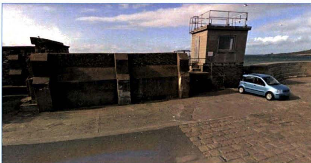
Plate 27: View looking West across the open space at the pier head, showing the buttressing that indicate the presence of former buildings, and the observation building that is built on top of earlier foundations.
