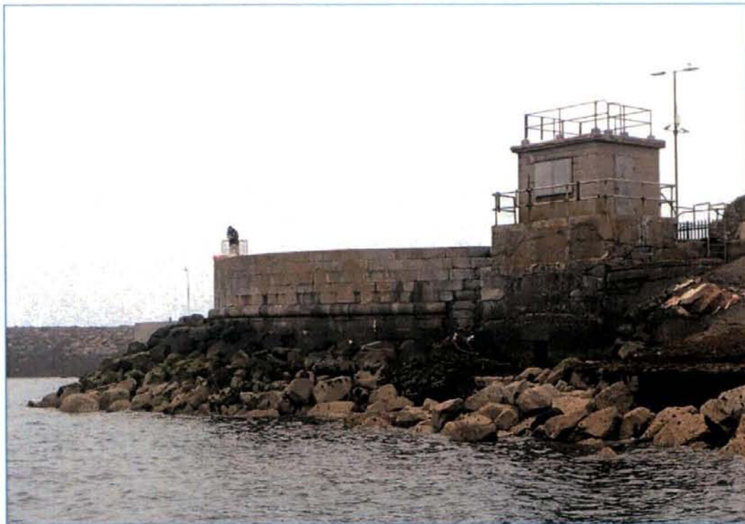
Plate 23: View from sea towards West Pier roundel, showing the rolled moulding at the base of the wave barrier. Picture includes the later observation building to the south (right) of the roundel.
