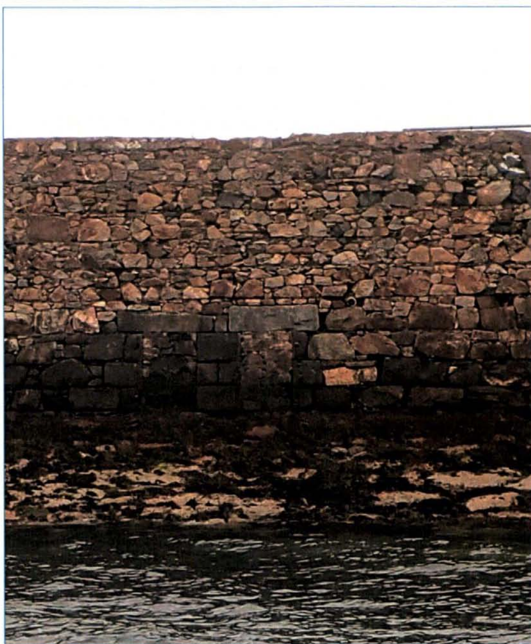
Plate 35: Detail of Plate 34 highlighting a pair of the lintelled culverts that have been blocked up.
