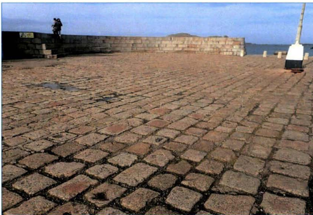
Plate 18: Granite cobbled surface of the pier head roundel.
