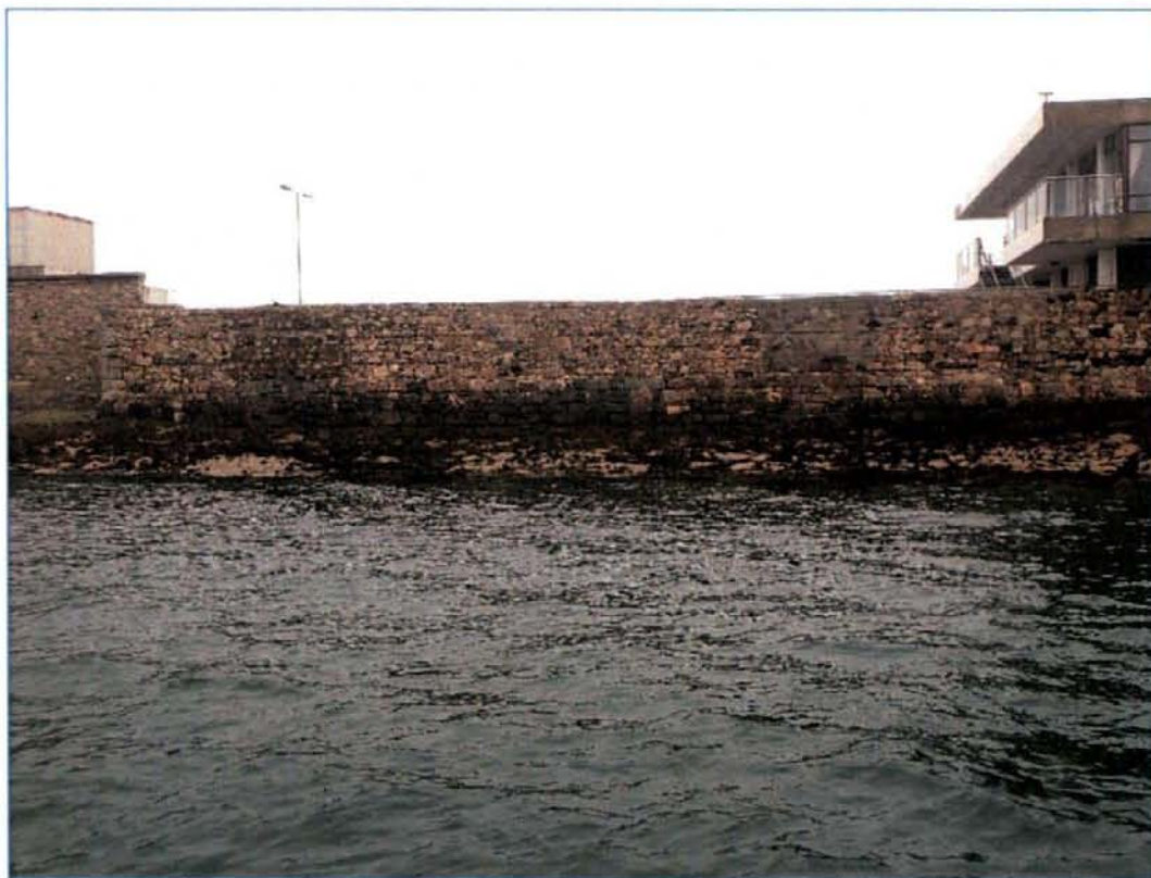
Plate 34: Second stone retaining wall with granite used as corner stones. This stretch also includes lintelled culverts that would have serviced the terrace of houses that formerly stood inside (east of) the retaining wall.
