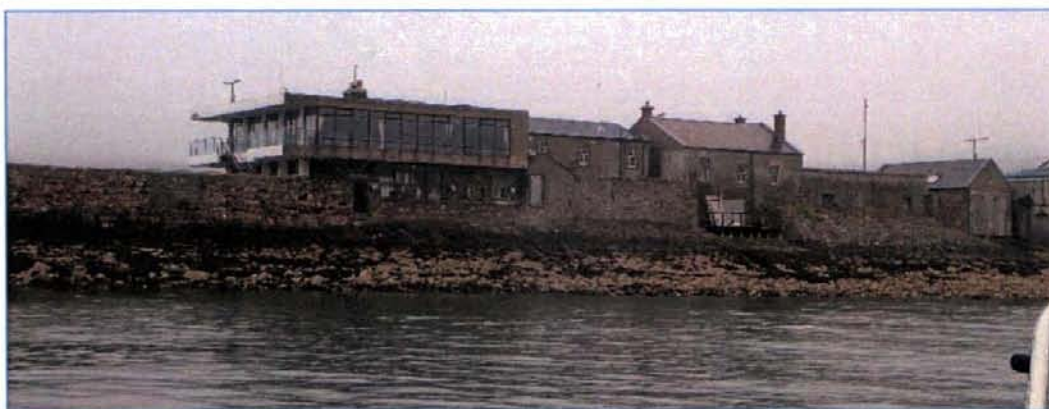
Plate 29: View from the sea showing the glacis that extends along the rear of the West Pier.
