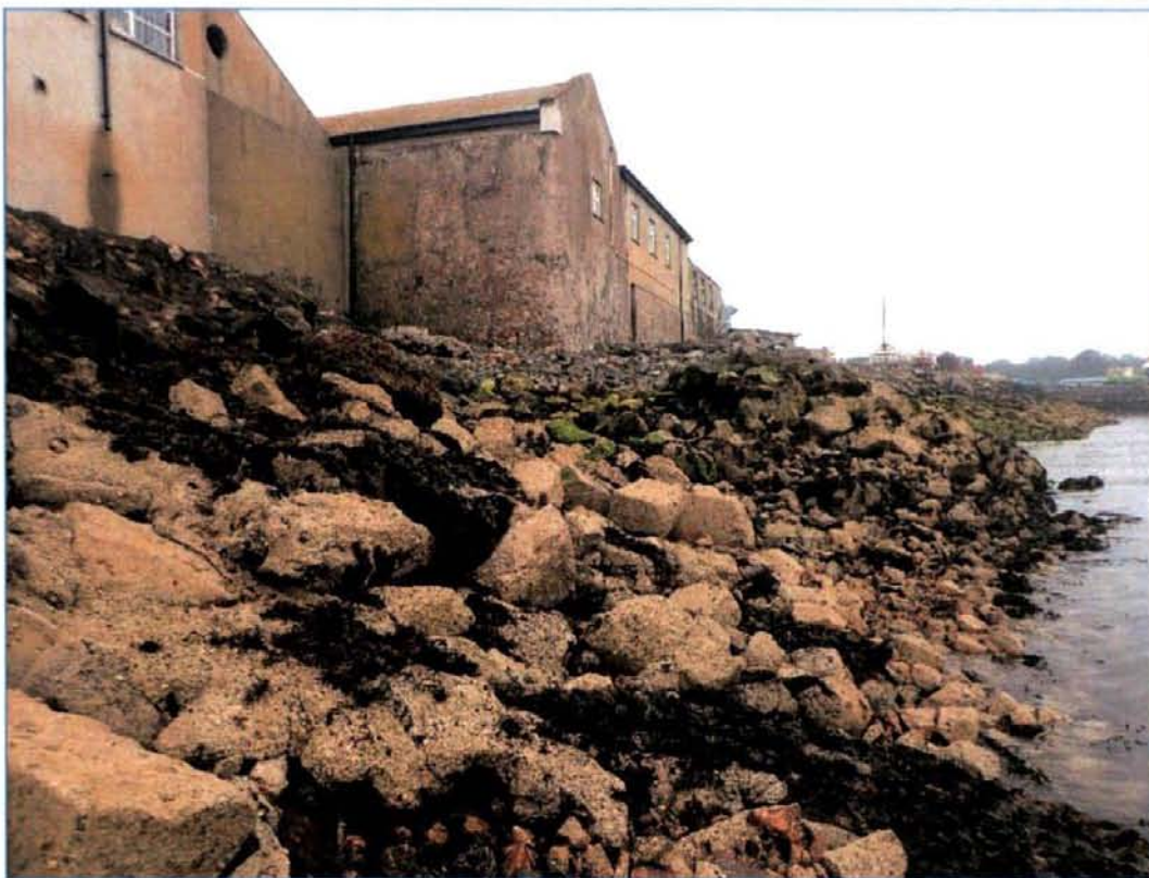
Plate 47: View looking South from the slipway at the coastguard slipway along rock armour that has been added, effectively burying the glacis.
