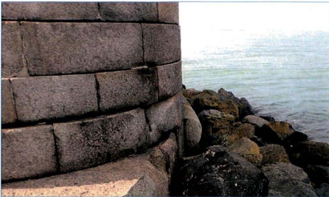
Plate 21: View focussed on rolled moulding at external base of West Pier roundel.
