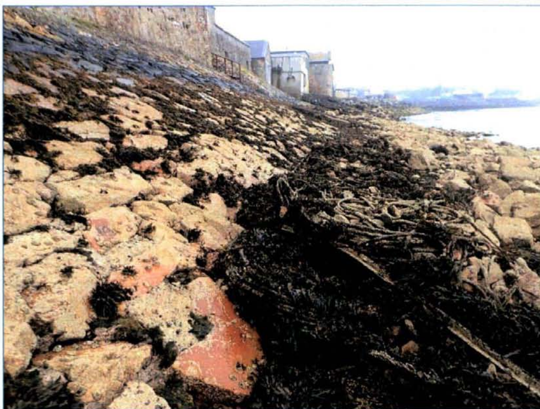
Plate 31: View looking South showing detail of stonework along glacis.
