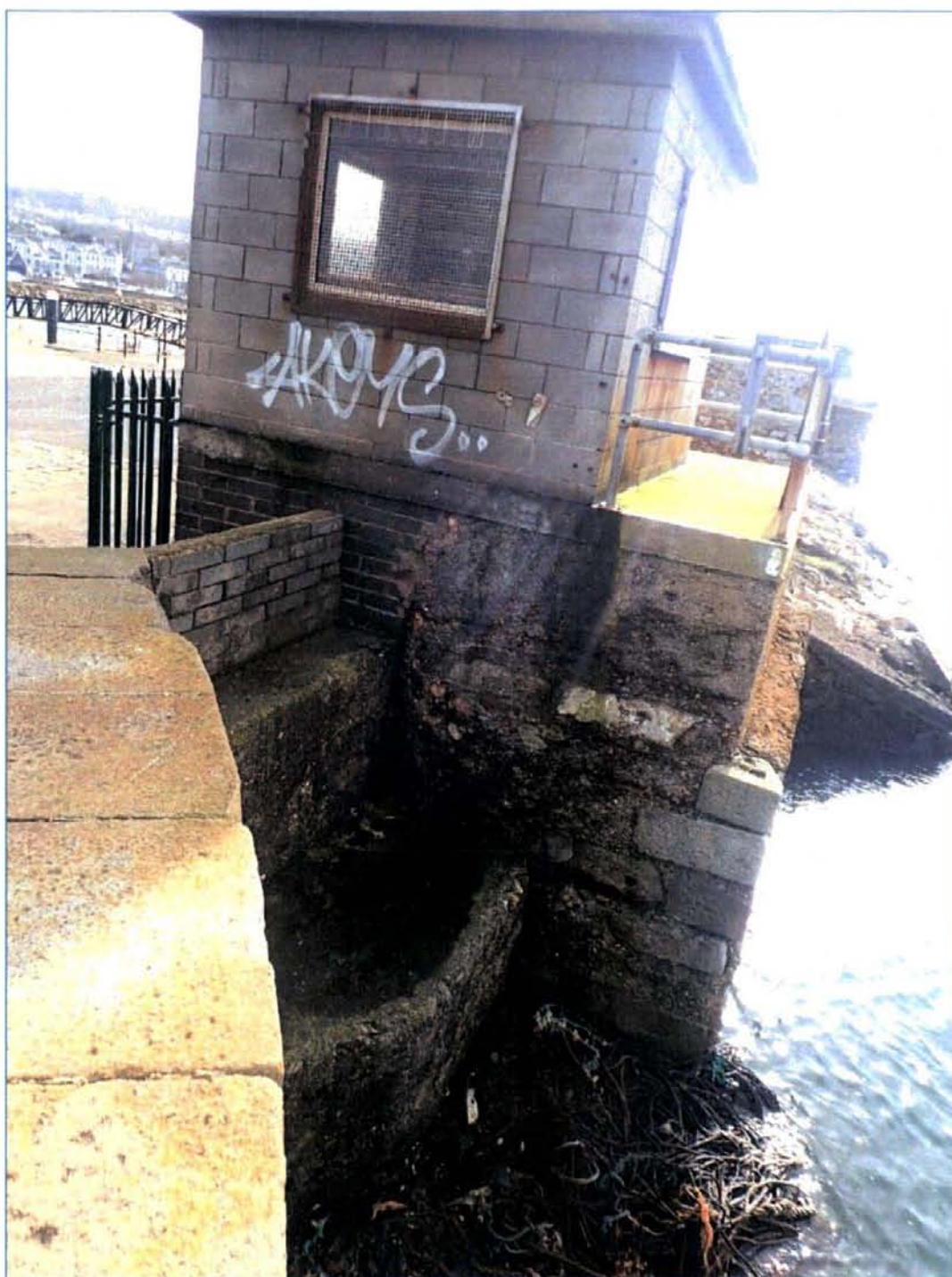
Plate 24: View looking South from roundel showing the non-uniform nature of the integration with the West Pier. The picture also shows the later observation building and its construction of earlier foundations.
