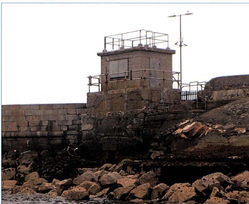
Plate 28: View from the sea highlighting the observation building and its squared concrete foundations standing on top of and earlier stone-and-concrete foundation.
